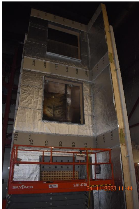
Photo No. 6 Cembrit boards mounted to the gap.
