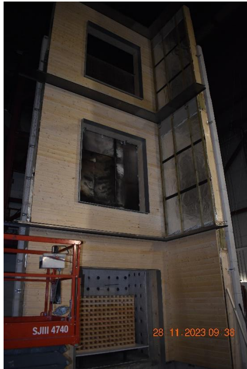
Photo No. 13 Horizontal cladding is being mounted.
