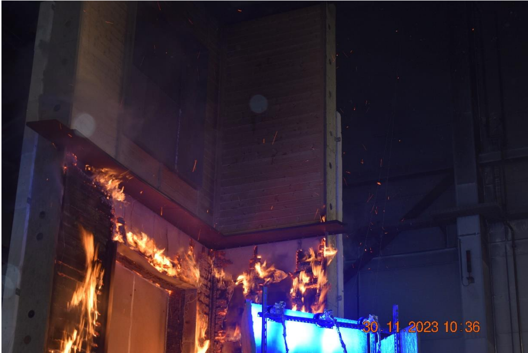
Photo No. 27 Test specimen 36 minutes into the test.
