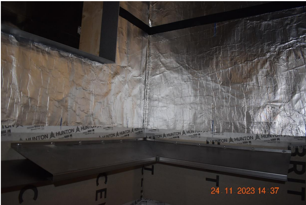
Photo No. 10 Flame deflectors are being mounted.
