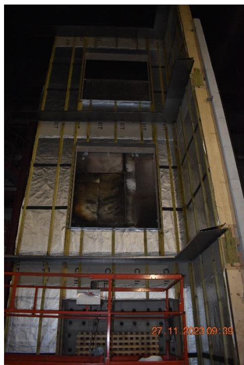
Photo No. 12 Vertical formworks have been mounted.
