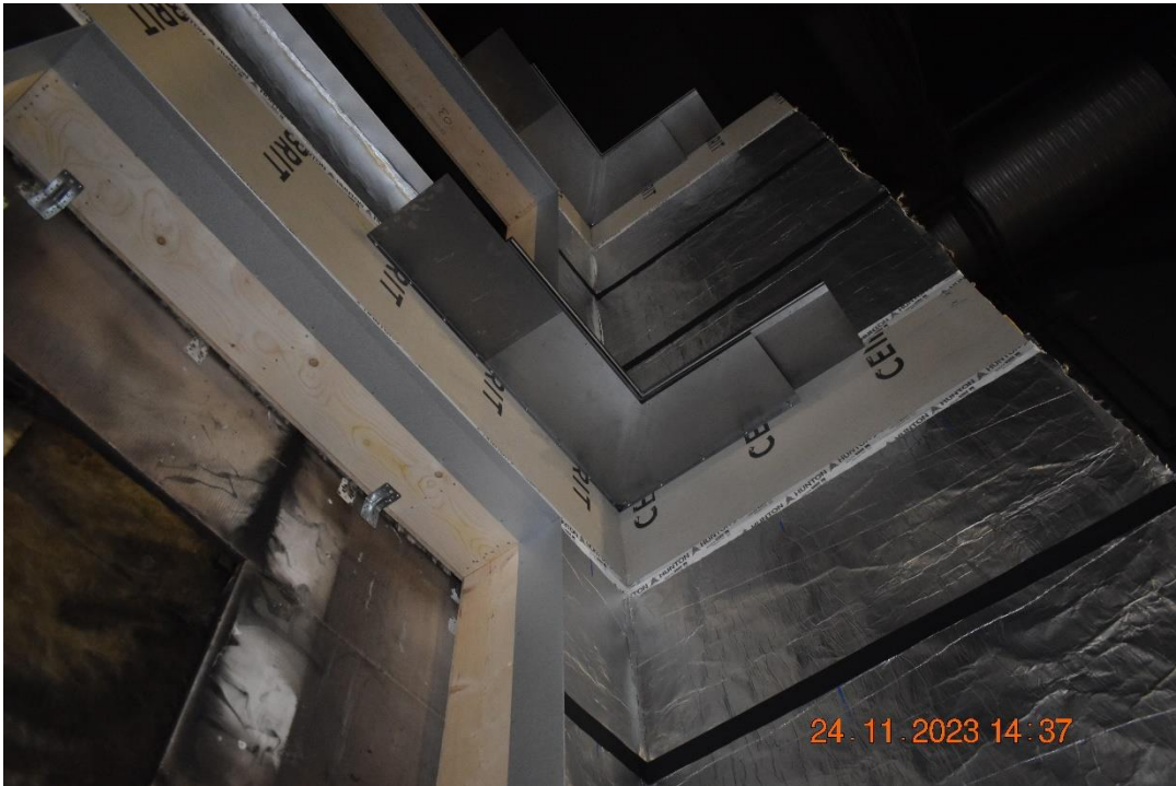
Photo No. 11 Corner flame deflectors have been mounted.
