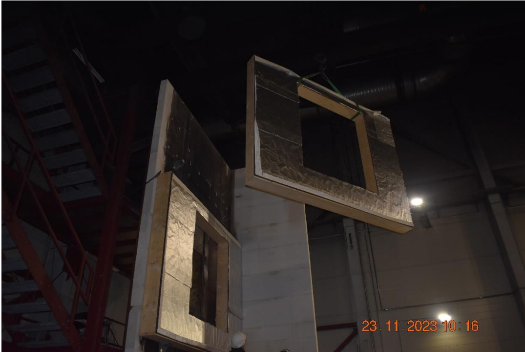
Photo No. 1 Prefabricated cassettes being mounted.
