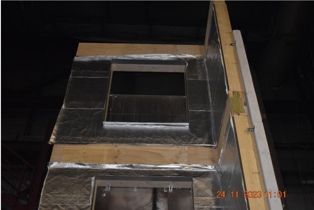
Photo No. 5 Membrane on the top of the windbreaker.
