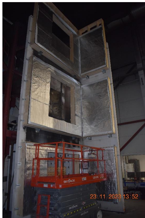
Photo No. 2 Fixing of prefabricated cassettes.
