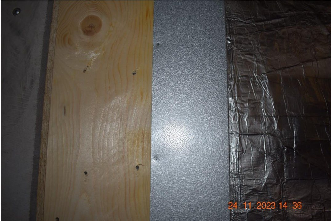
Photo No. 9 Profiles around windows and fire chamber are being installed.
