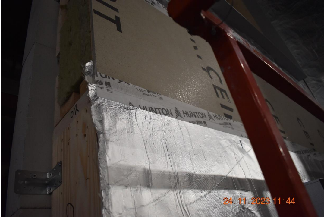
Photo No. 7 Hunton Tescon Vana tape to connect the membrane to Cembrit board.
