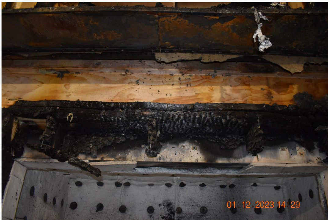
Photo No. 32 Test specimen after the test. Detailed photo of the top of fire chamber.
