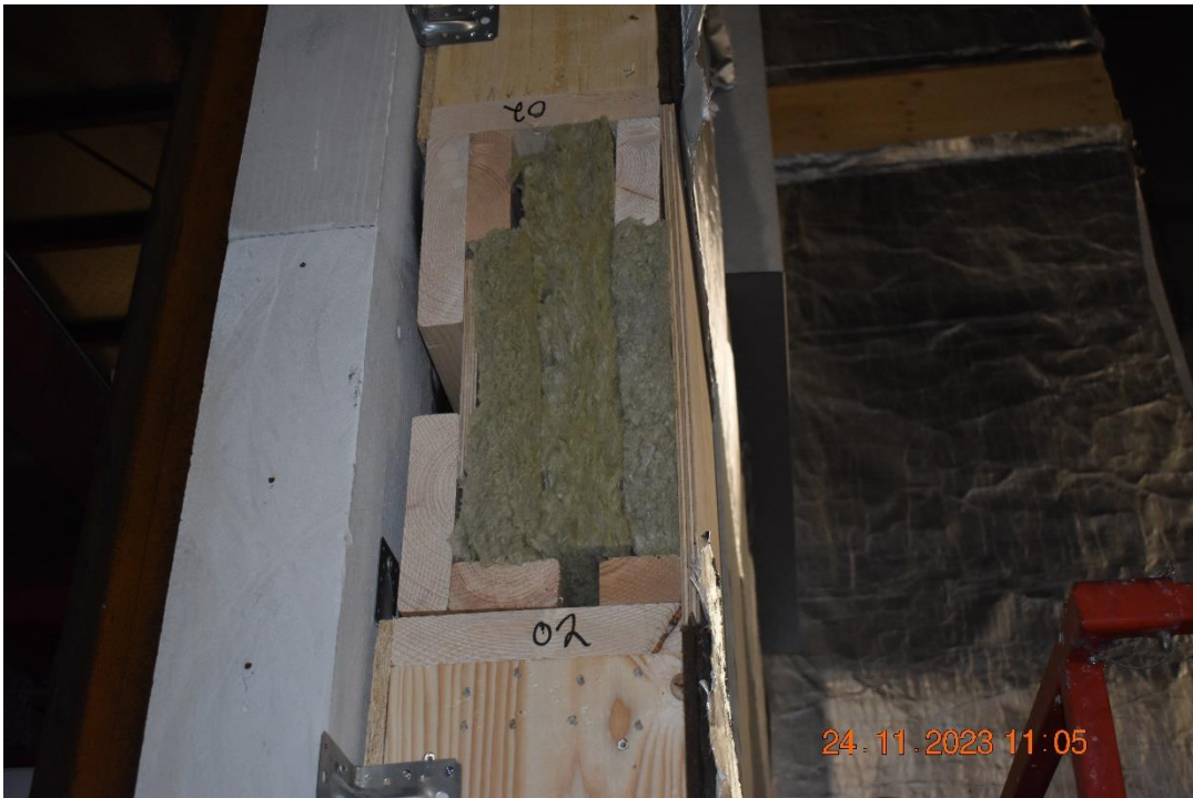
Photo No. 4 Insulation in the gap.
